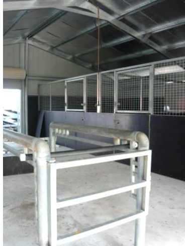
Figure 1: Our purpose-built equine facility and crush
